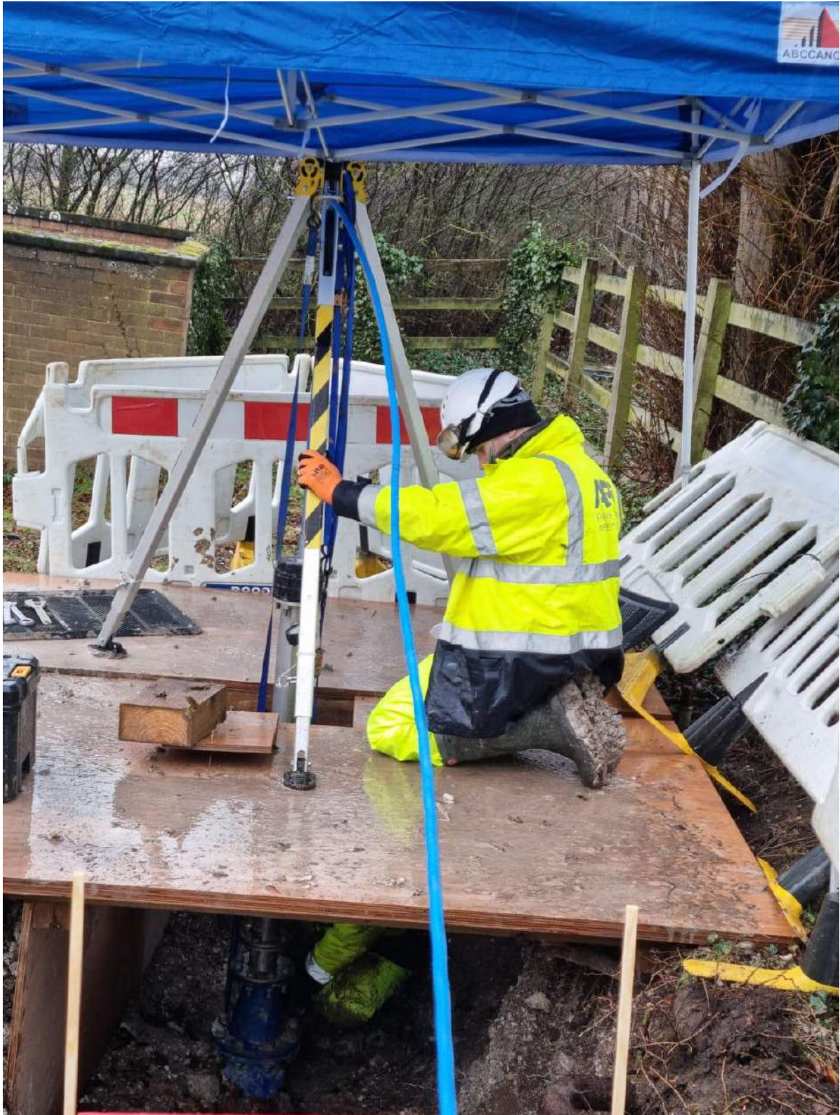
System site set up on a temporary excavation working platform required
